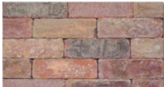
No Mortar Joint (Dry-Stacked)
